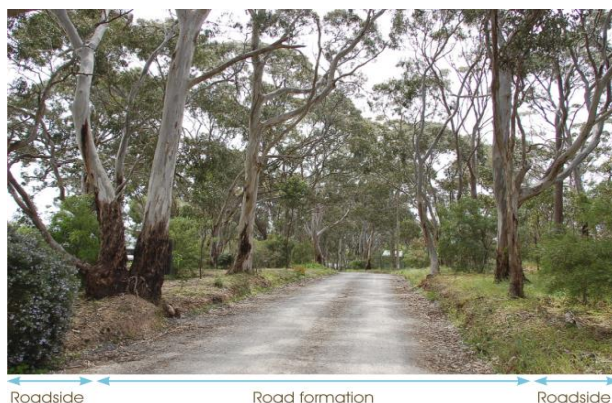
Example of a road reserve showing road formation and roadside
