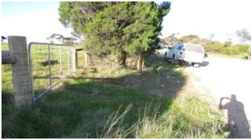
Poor driveway sight clearance
