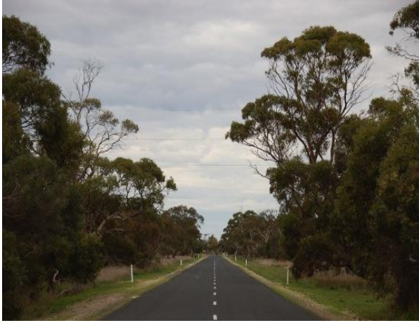
New Sealed Road
