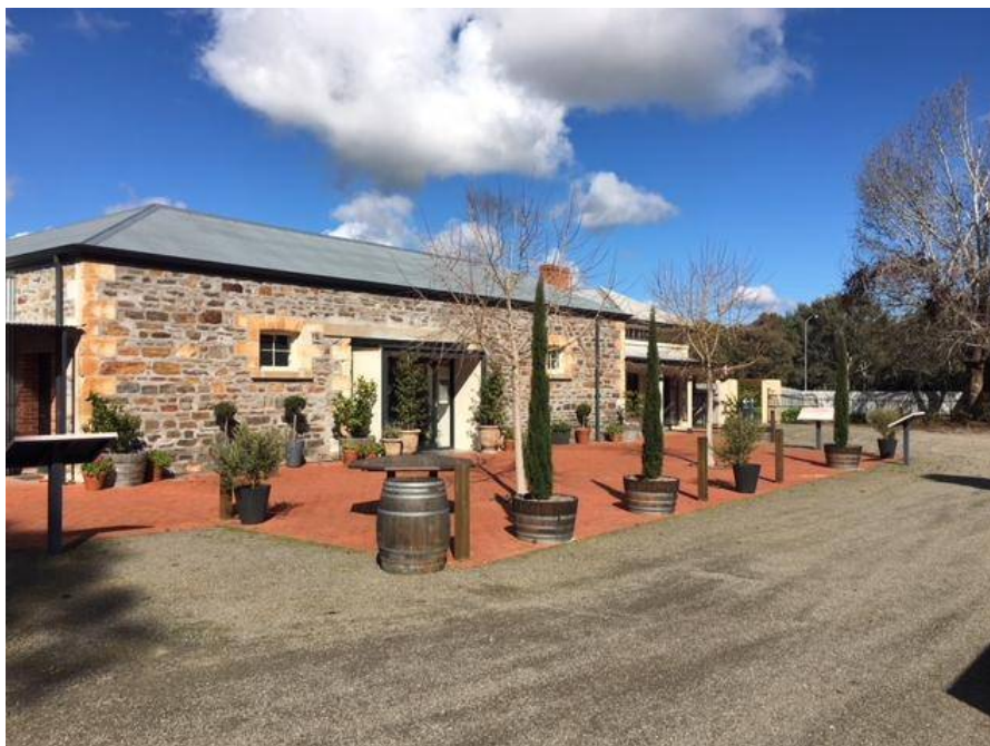
Photo 3: The existing cellar door and office buildings in the former stables building
