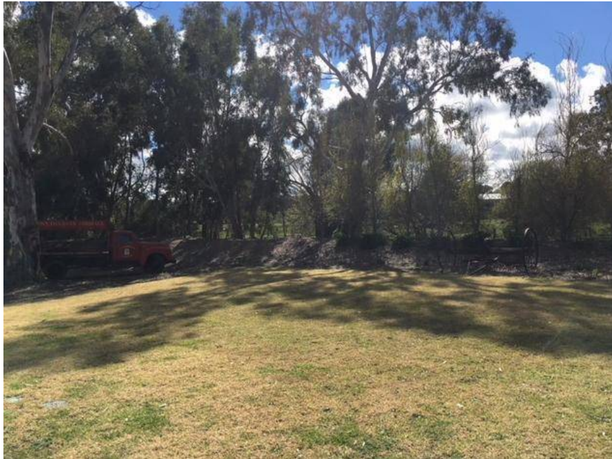
Photo 4: The levee adjacent to the Onkaparinga River for flood protection
