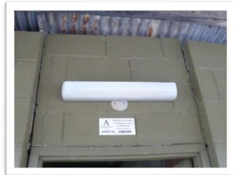
More cracks in the storeroom.
