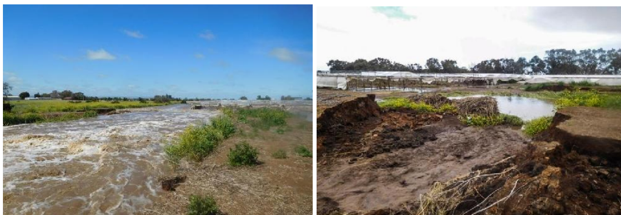
Figure 3.1 Levee breach during 2016 flood event
