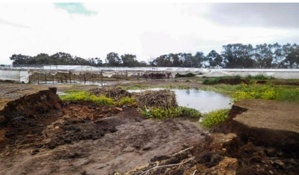
Levee bank failure during 2016 flood event resulting in flooding of horticultural areas.
