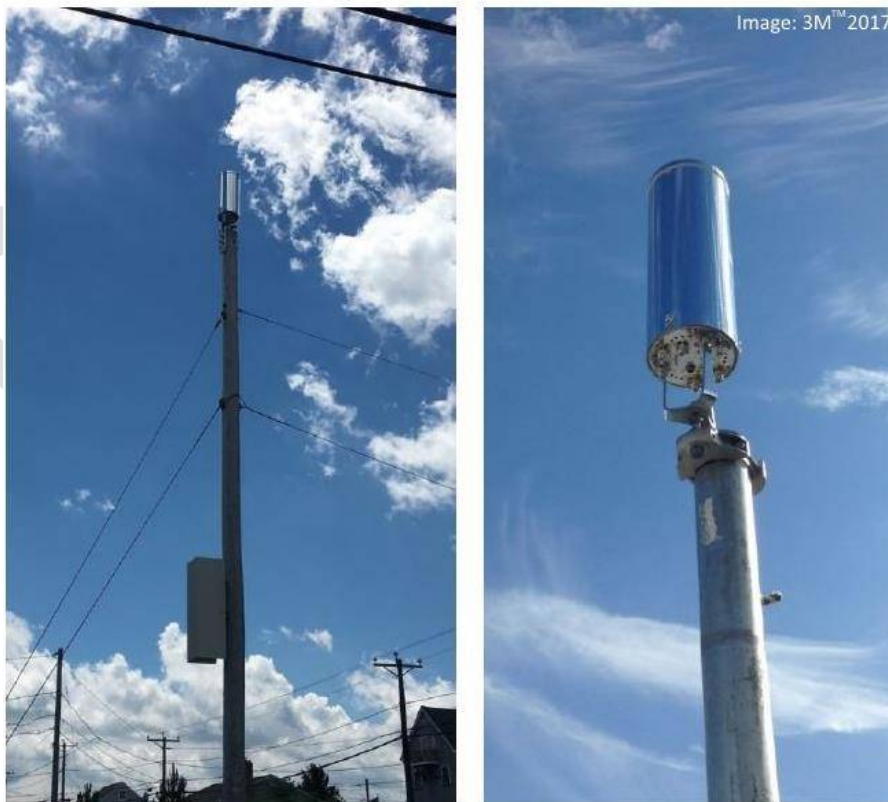
Figure 6: Reflective wrap installed on antennae to reflect background and respond to changing light conditions
