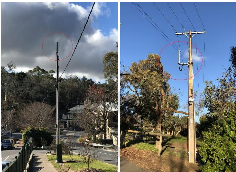
Figure 1 & 2: Current 4G installations with omni antenna on utility pole and ground based enclosure (Aldgate and Bridgewater installation)
