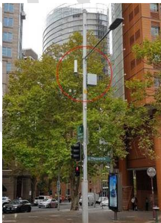
Figure 3: Current 4G installations using a “Koala” equipment enclosure on the pole (no ground based cabinet)
