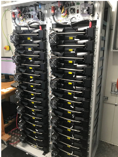
Figure 3: LG Chem battery rack
