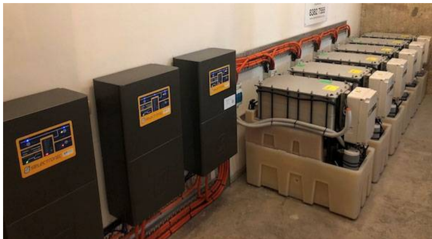
Figure 2: Redflow install - Darling Building
