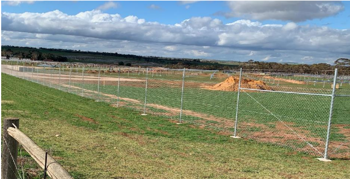
Fig.20. Typical solar farm perimeter fence (Approx. 2.3m high) source: Mannum Solar Farm
