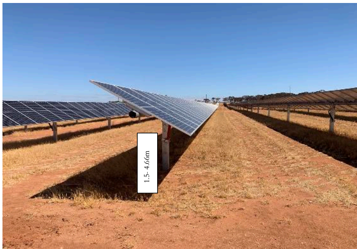
Fig.12. Example of a Single Axis Solar PV Array (Source: Tetris, Mannum solar farm)
