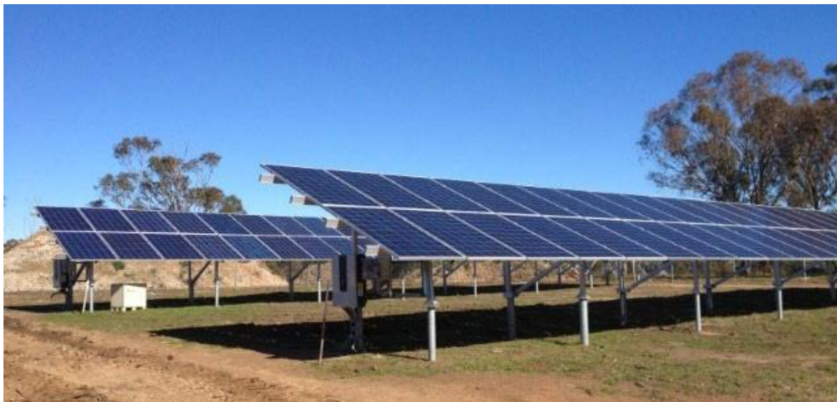
Fig.1. Example Solar PV Array – screw mounted
