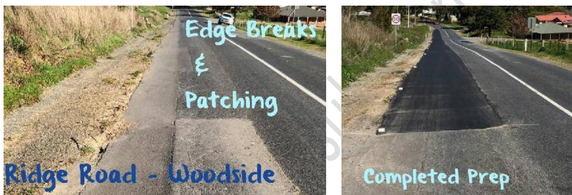
Woodside – Targeted Pavement Works – Before and After
