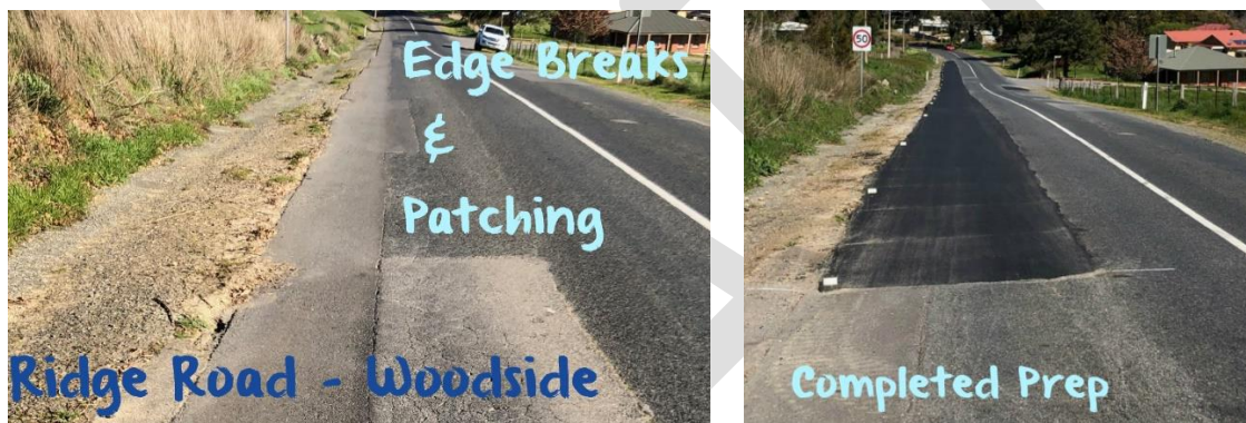
Woodside – Targeted Pavement Works – Before and After
