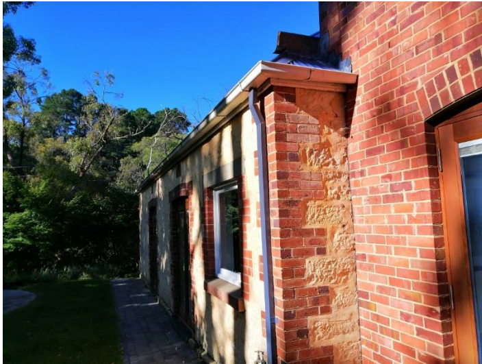
2. Photo showing gutters and timber that require replacing (West view)
