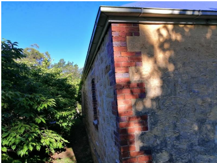
3. Photo showing gutters and timber that require replacing (North view)
