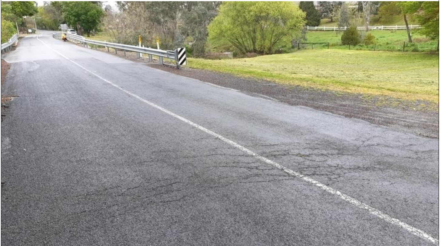
Image Number: 8 Image Name: BR004_008 Description: View of minor Cracking on wearing surface on bridge approach 1.
