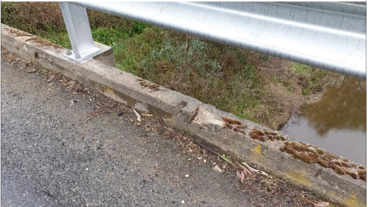
Image Number: 25 Image Name: BR004_025 Description: View of moderate cracking and spalling on kerb on kerb 2.
