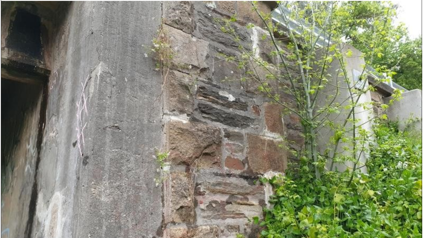
Image Number: 63 Image Name: BR004_063 Description: View of typical cracking through masonry retaining wall on retaining wall 2.
