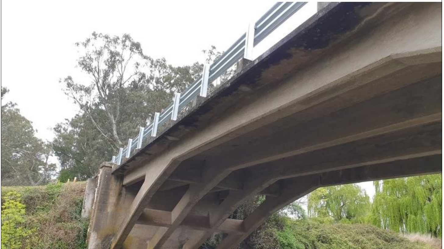
Image Number: 42 Image Name: BR004_042 Description: Additional view of moisture staining throughout deck edges on deck slab 1.
