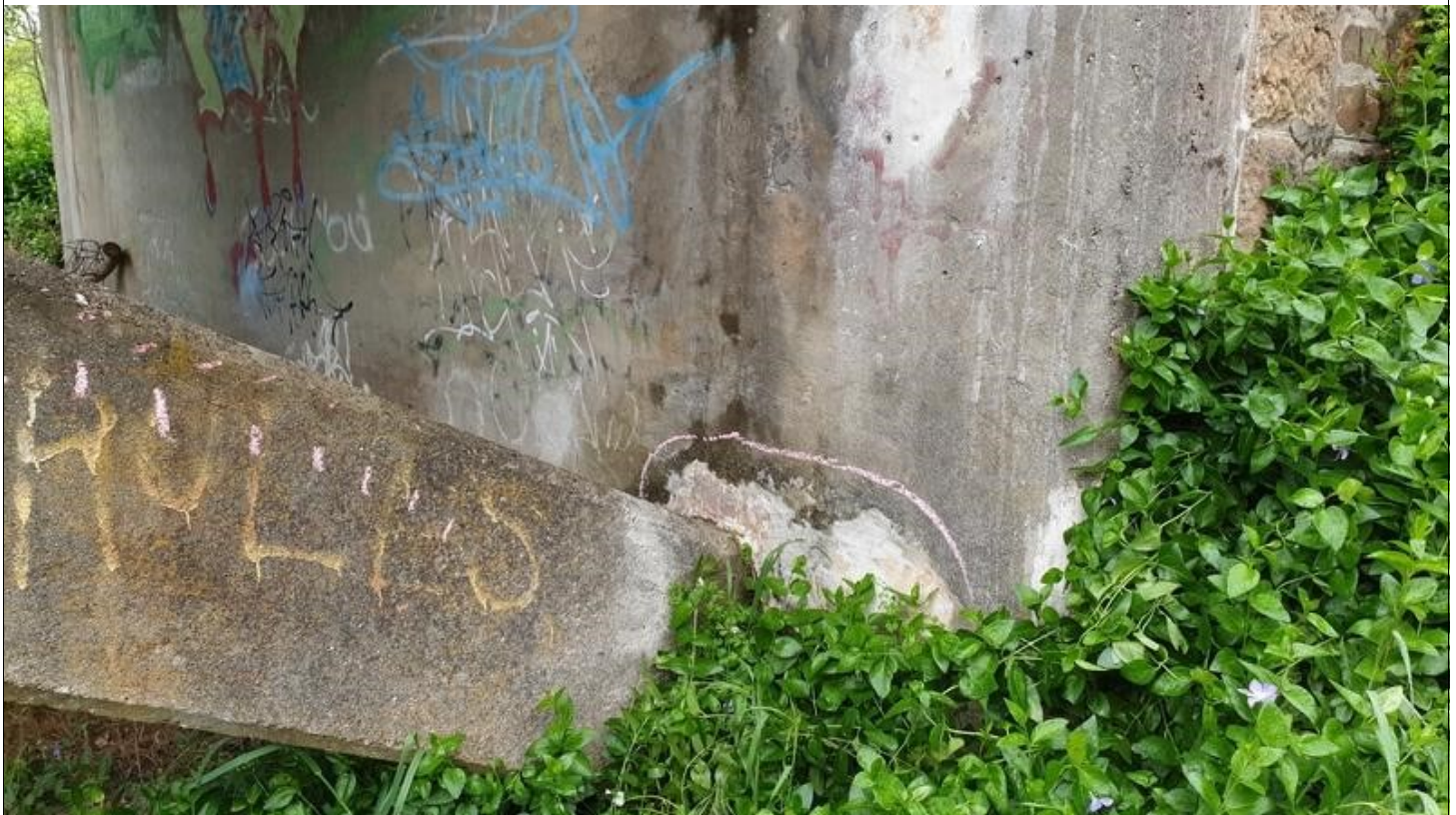
Image Number: 60 Image Name: BR004_060 Description: View of efflorescence above column 4 on abutment 1.
