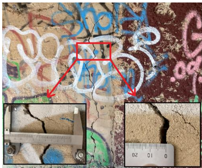
Figure 2.31 4 mm wide crack on the left-hand side of abutment 2 – the spacing of anchorage bolts measured as 90 mm
