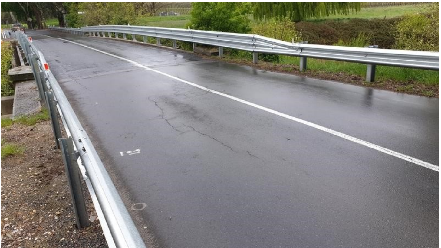
Image Number: 31 Image Name: BR004_031 Description: View of minor cracking on wearing surface on bridge approach 1.
