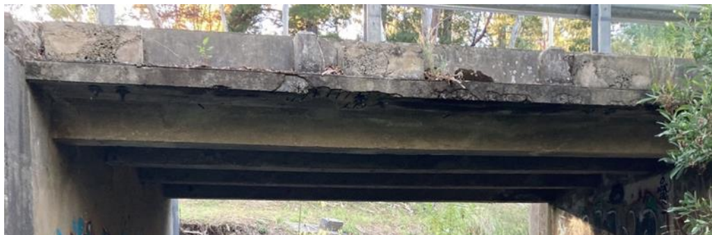
Figure 2.9 Abrasion and delamination on the outer face of the right-hand side kerb
