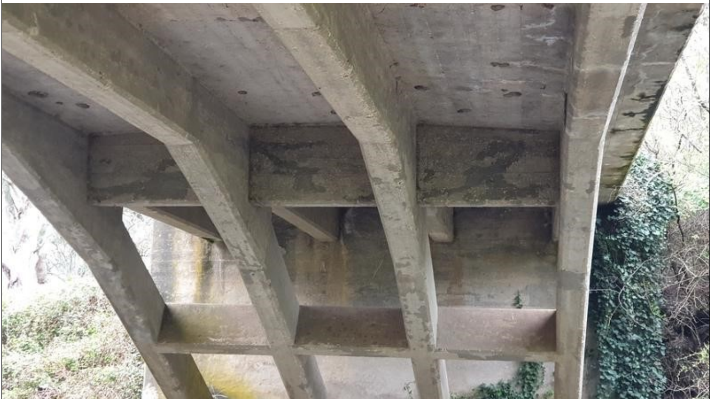
Image Number: 48 Image Name: BR004_048 Description: View of cross bracing.
