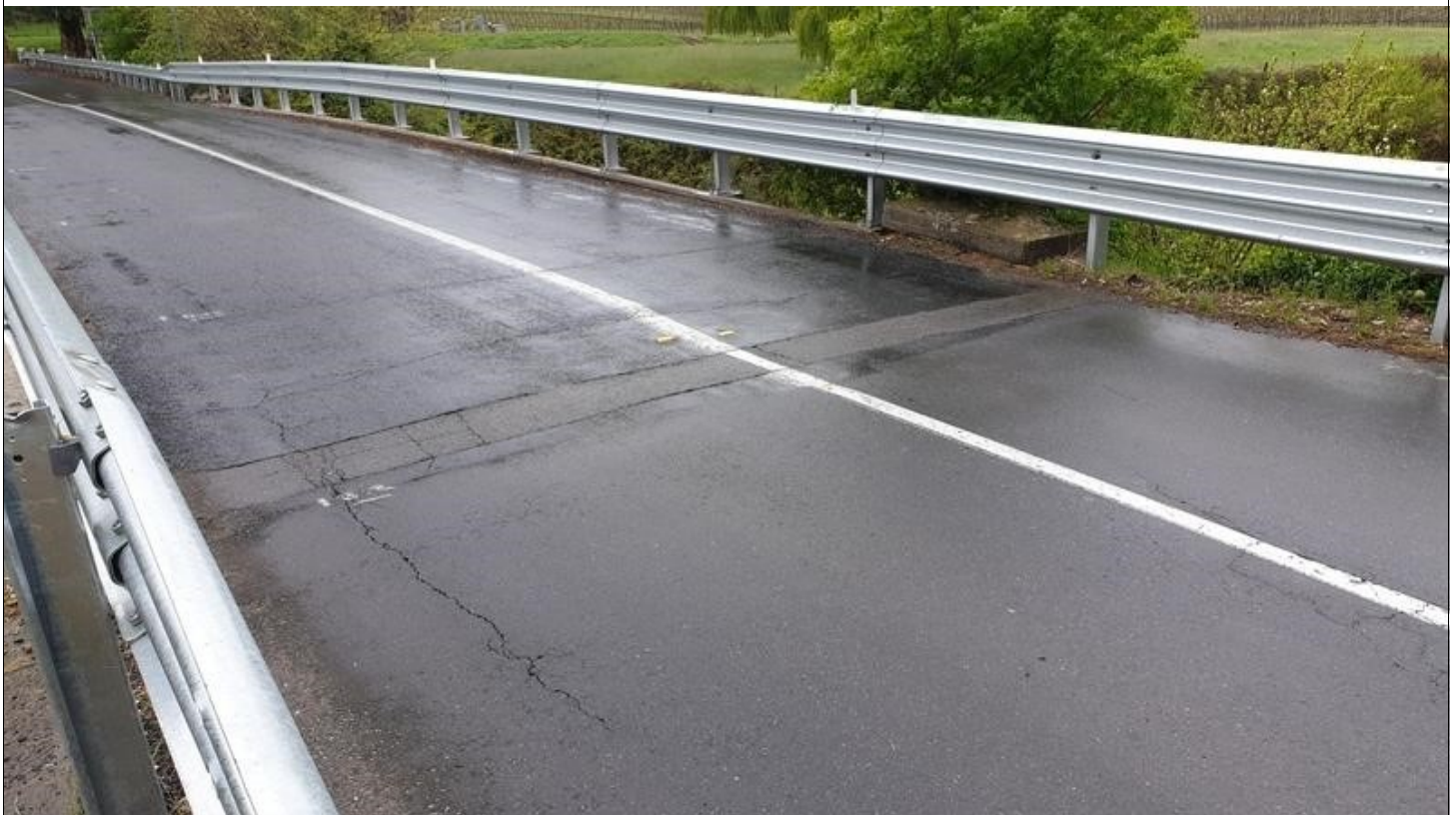
Image Number: 32 Image Name: BR004_032 Description: View of longitudinal cracking on bridge approach 1.
