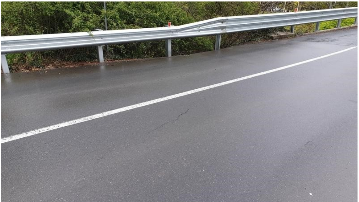
Image Number: 9 Image Name: BR004_009 Description: Additional view of minor Cracking on wearing surface on bridge approach 1.
