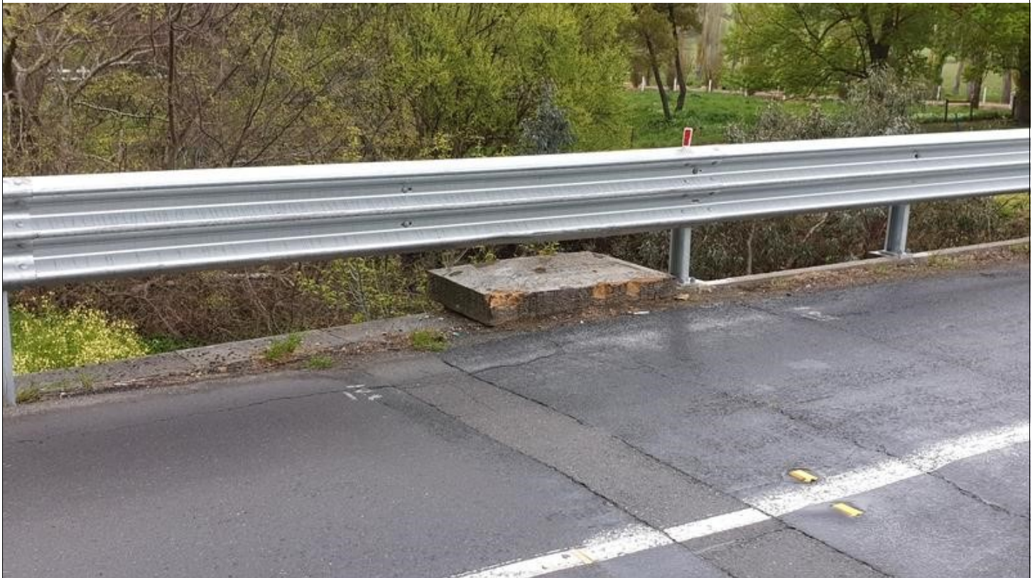
Image Number: 26 Image Name: BR004_026 Description: Additional view of moderate cracking and spalling on kerb on kerb 2.
