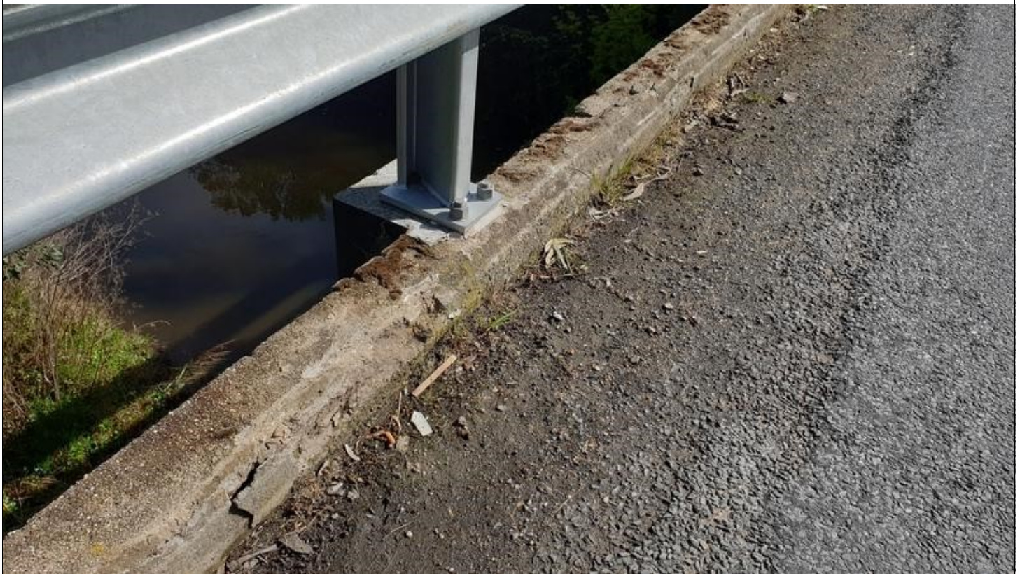
Image Number: 27 Image Name: BR004_027 Description: Additional view of moderate cracking and spalling on kerb on kerb 2.
