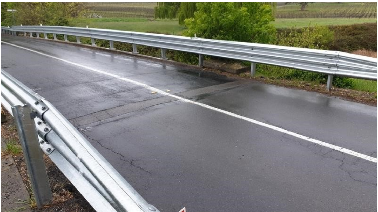
Image Number: 29 Image Name: BR004_029 Description: View of pourable joint seal 1.
