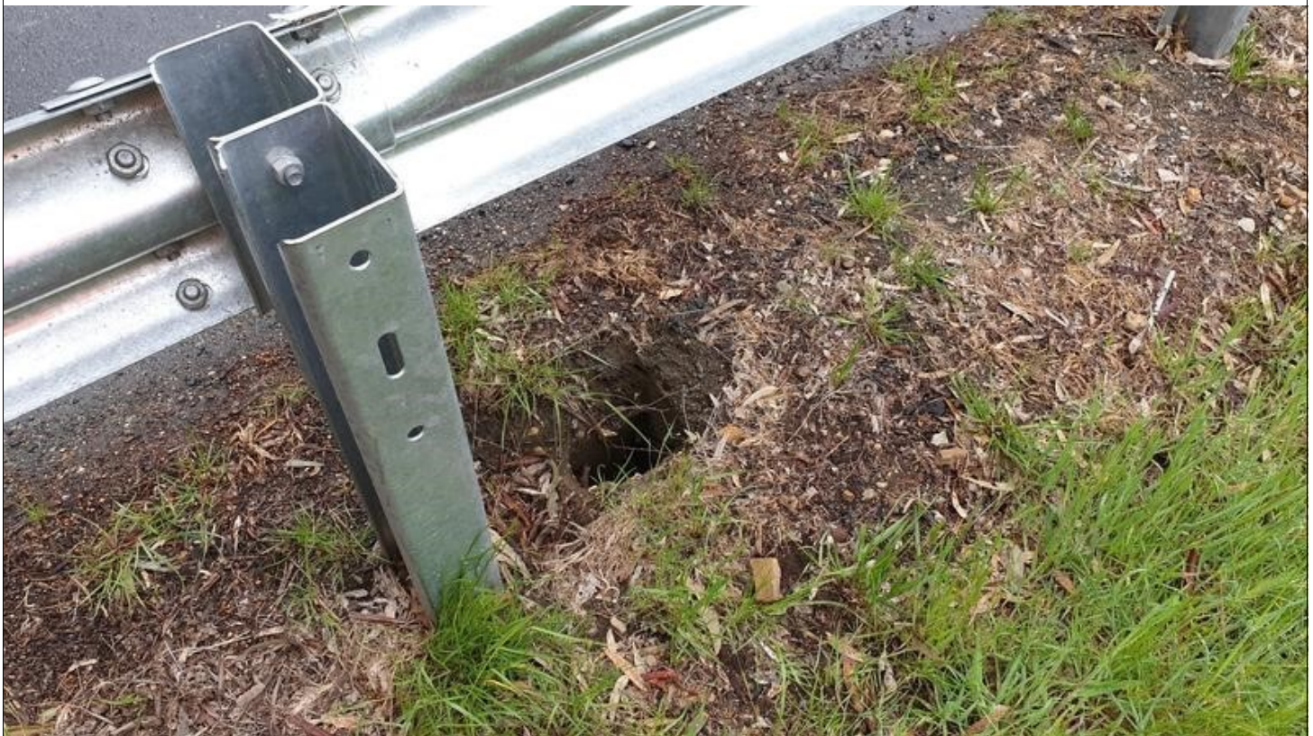
Image Number: 30 Image Name: BR004_030 Description: View of hole left from former barrier post (300mm) deep on guardrail 1.
