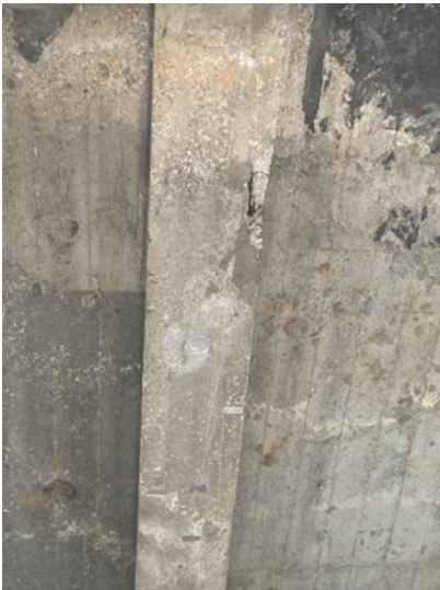
Figure 2.5 Severe concrete chipping and exposed reinforcement on the right-hand side edge of girder 3, located at mid-span
