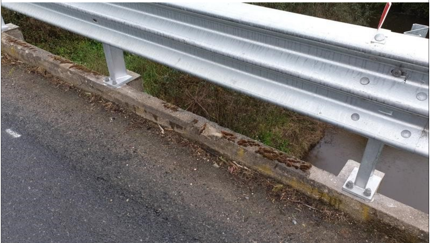
Image Number: 17 1. Image Name: BR004_017 Description: View of minor spalling and cracking along kerb with reinforcement exposed on kerb 1.
