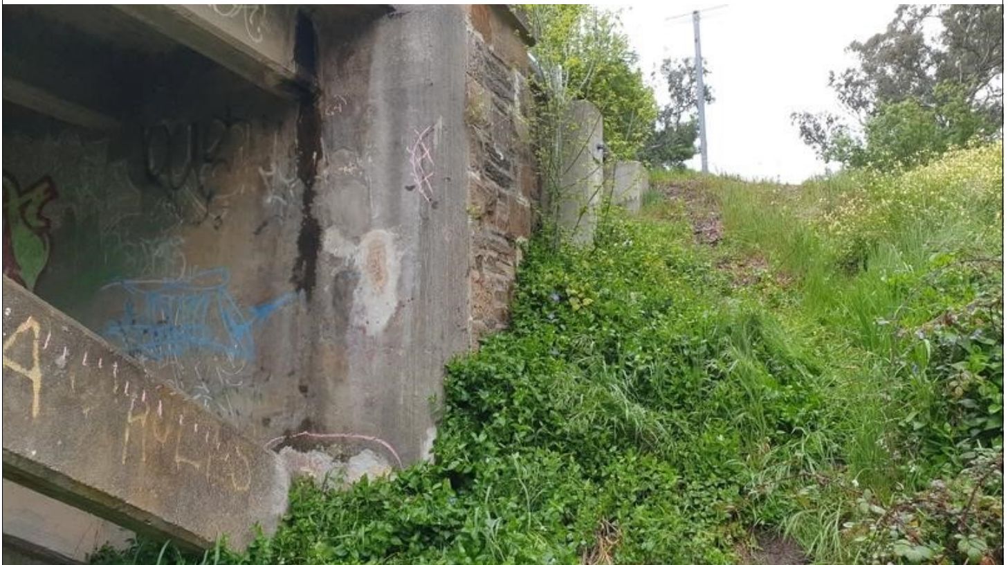
Image Number: 64 Image Name: BR004_064 Description: View of vegetation encroaching retaining wall on retaining wall 2.
