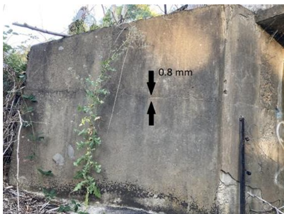
Figure 2.10 Moderate 0.8 mm wide horizontal crack extending across wingwall 2 left-hand side
