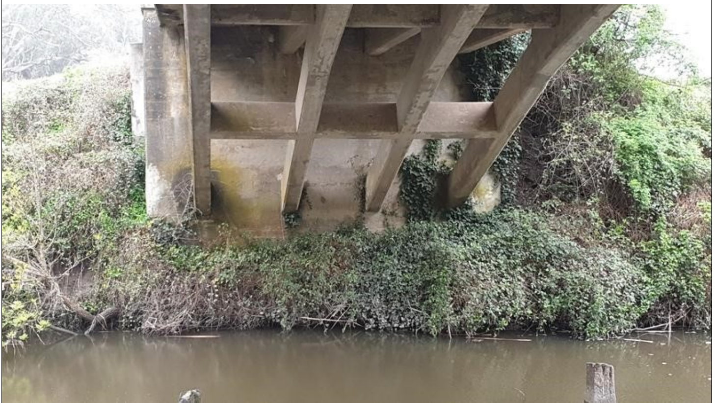
Image Number: 37 Image Name: BR004_037 Description: View of vegetation encroaching component on abutment 1.
