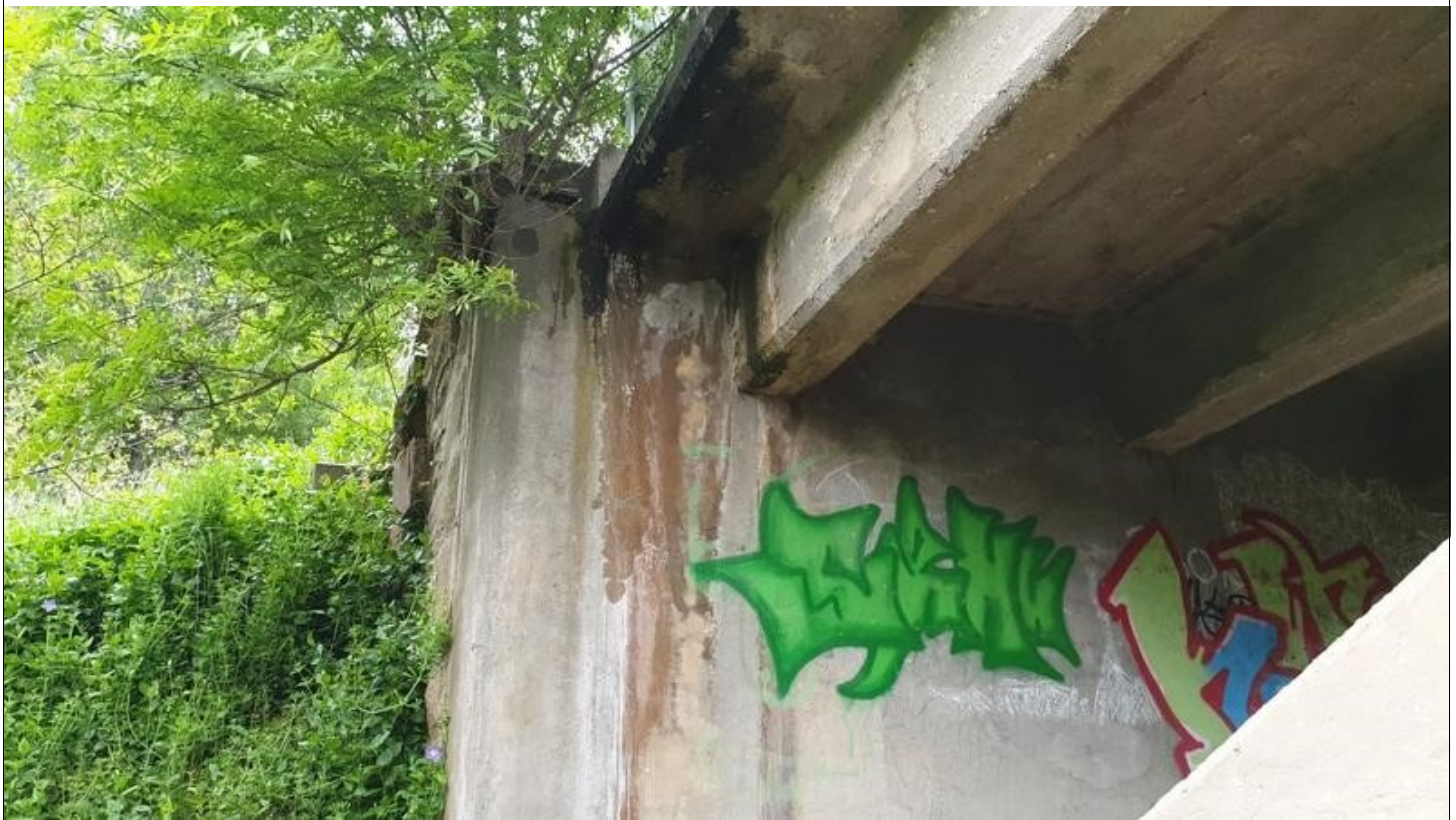
Image Number: 61 Image Name: BR004_061 Description: View of moisture staining under girder 1 on abutment 1.
