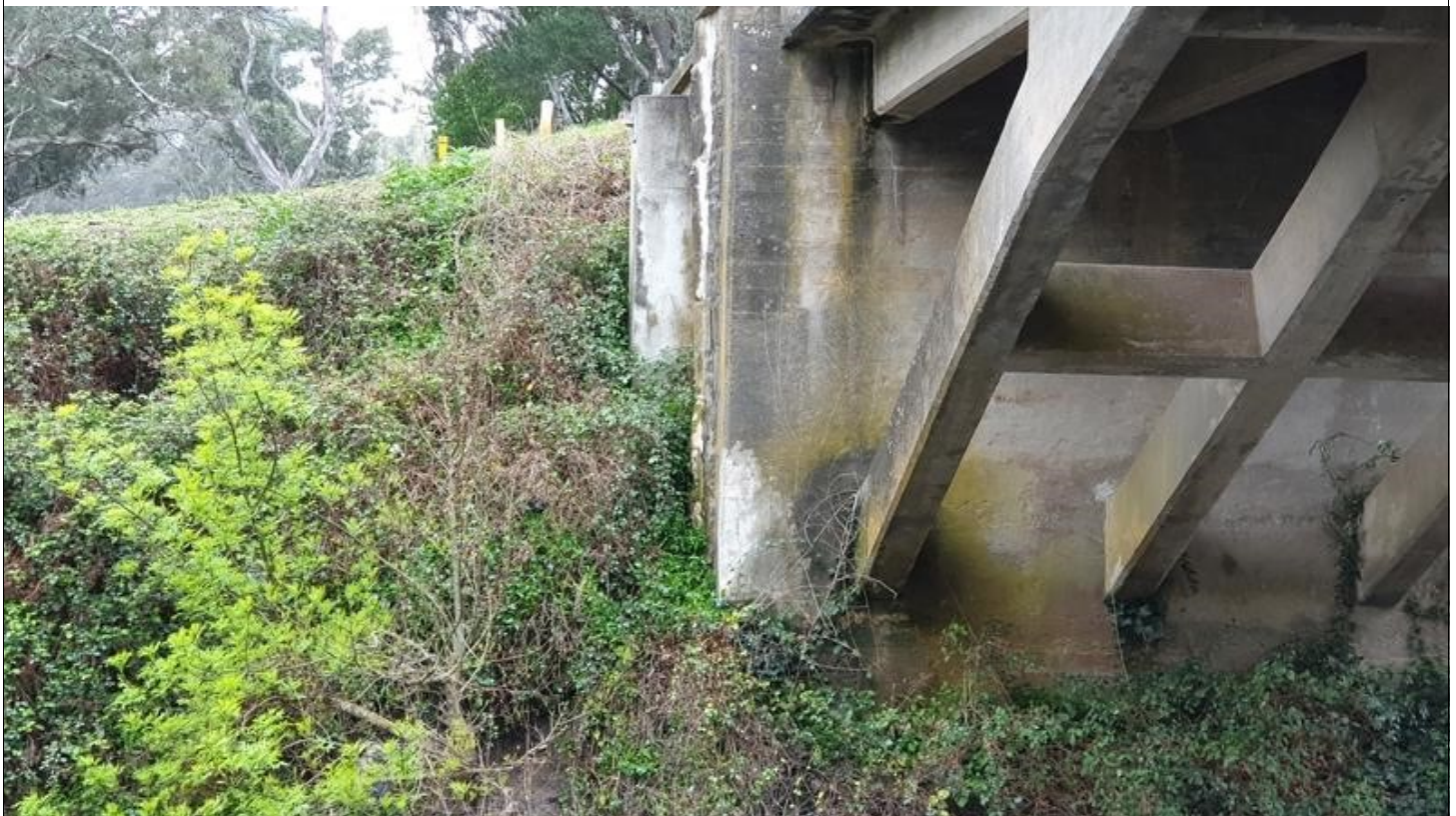
Image Number: 40 Image Name: BR004_040 Description: View of vegetation encroaching componen on retaining wall 2.
