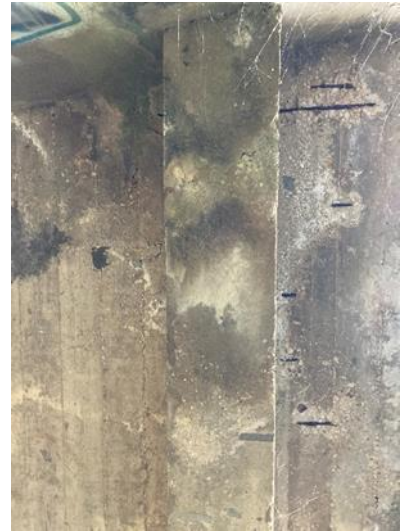
Figure 2.4 Severe spalling and exposed reinforcement near end 2 of girder 1
