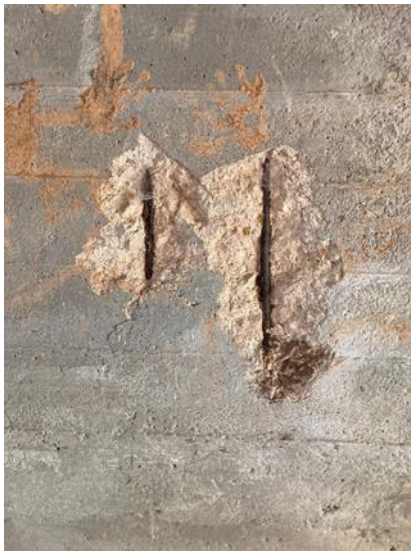
Figure 2.20 Spalling and exposed reinforcement on abutment 2 – box culvert section
