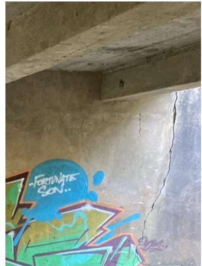
Figure 2.7 Extreme 5 mm wide vertical crack on left-hand side of abutment 1
