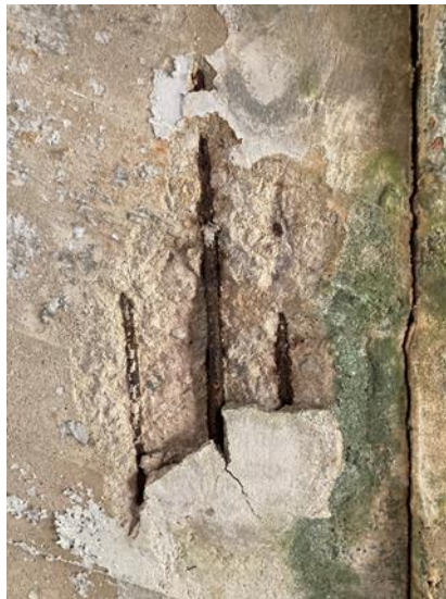
Figure 2.21 Spalling and exposed reinforcement on soffit of box culvert section, near the centreline
