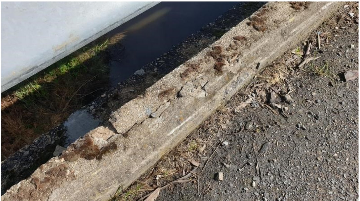
Image Number: 28 Image Name: BR004_028 Description: Additional view of moderate cracking and spalling on kerb on kerb 2.
