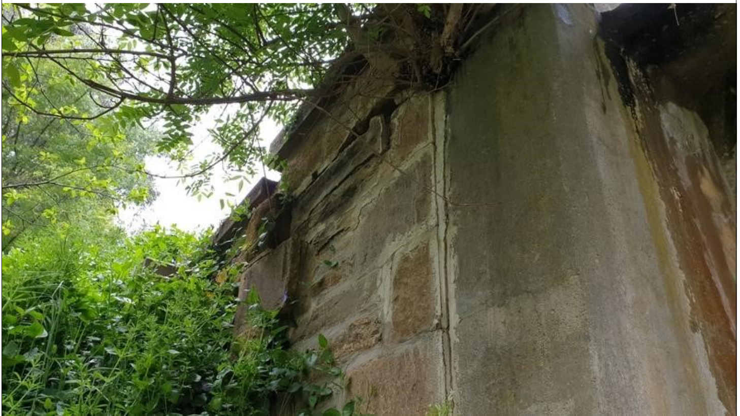
Image Number: 57 Image Name: BR004_057 encroaching component on retaining wall 1.
