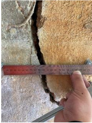
Figure 2.25 Installed anchorage bolts spacing, right-hand side of abutment 2 – 205 mm
