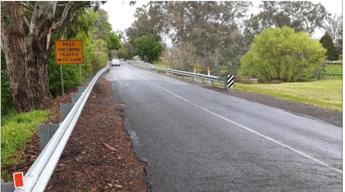
Image Number: 10 Image Name: BR004_010 Description: View of edge of approach surface breaking away on bridge approach 1.
