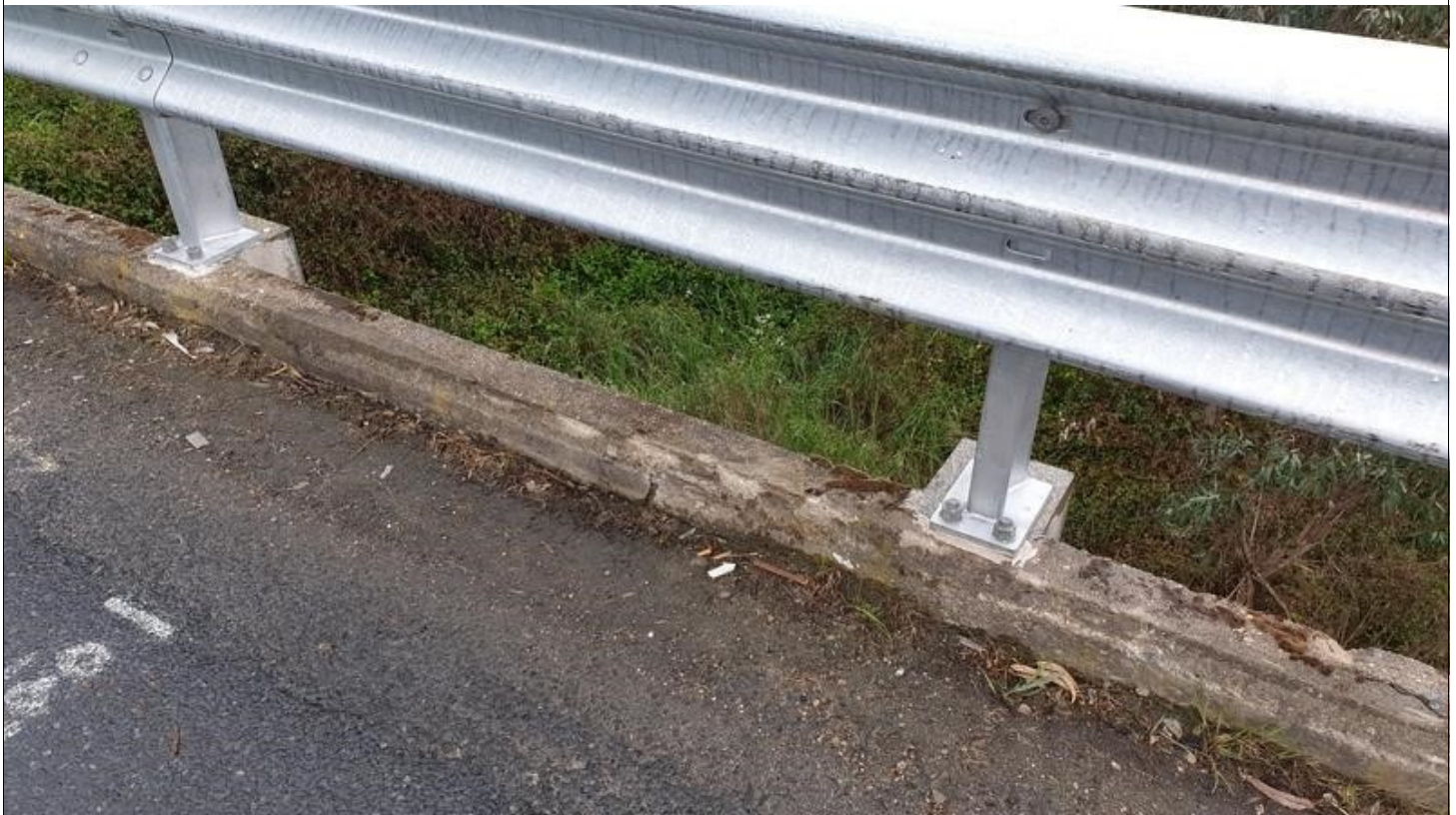
Image Number: 18 exposed on kerb 1. Image Name: BR004_018 Description: Additional view of minor spalling and cracking along kerb with reinforcement exposed on kerb 1.
