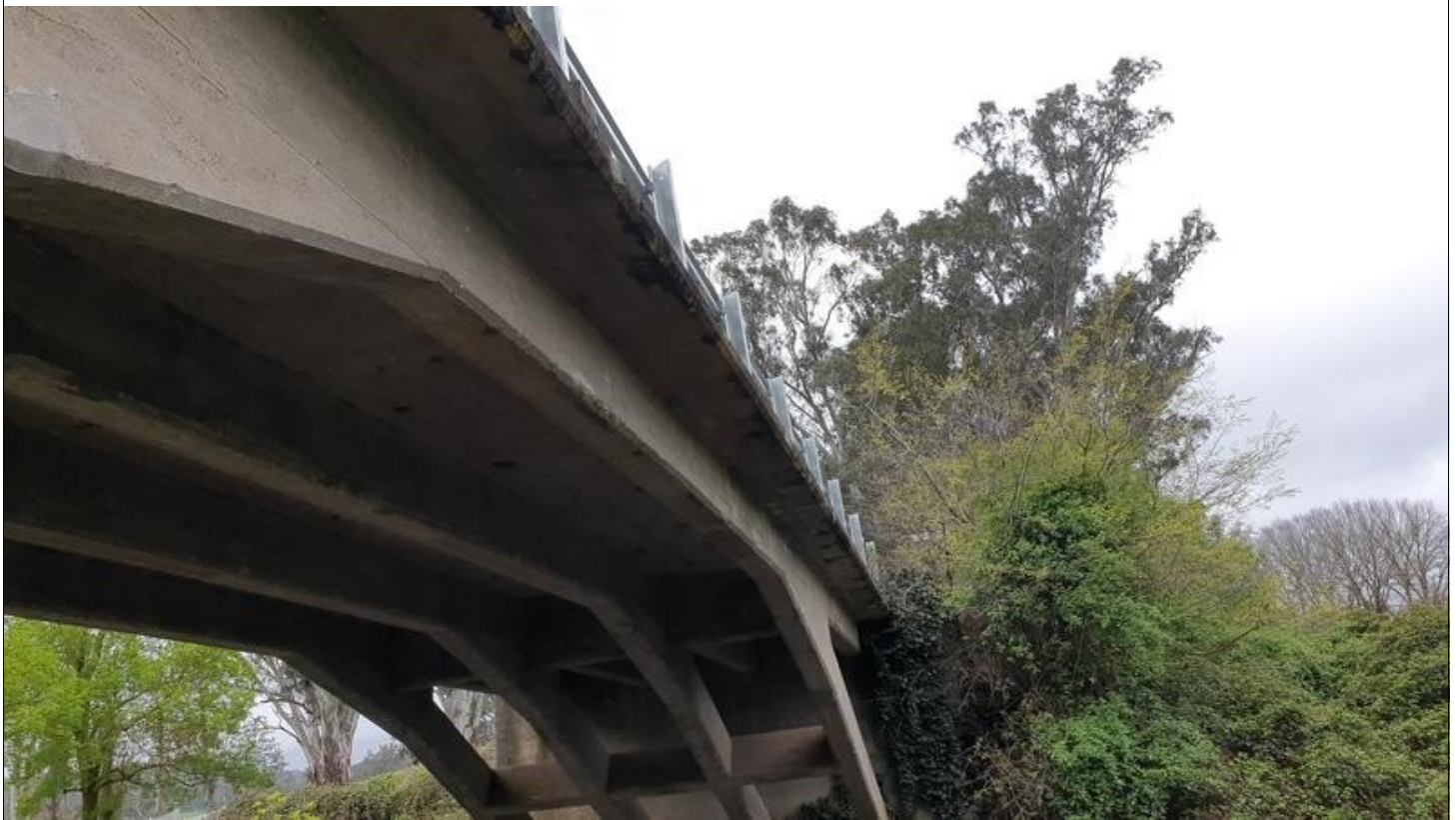
Image Number: 43 Image Name: BR004_043 Description: Additional view of moisture staining throughout deck edges on deck slab 1.
