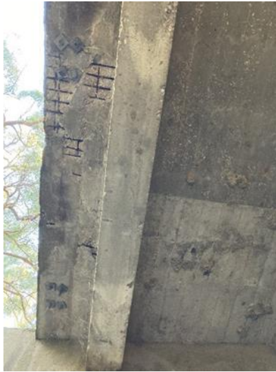
Figure 2.3 Severe spalling and exposed reinforcement near end 1 of girder 4
