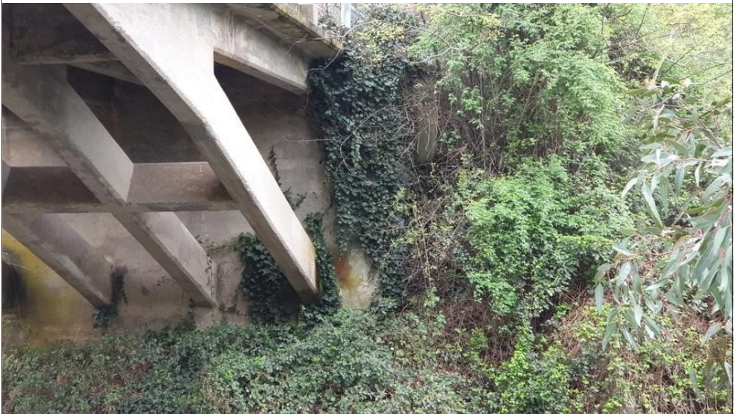
Image Number: 35 Image Name: BR004_035 Description: View of vegetation encroaching component on retaining wall 1.
