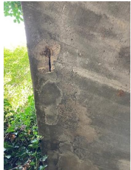
Figure 2.22 Spalling and exposed reinforcement on soffit of box culvert section, near the left-hand side edge
