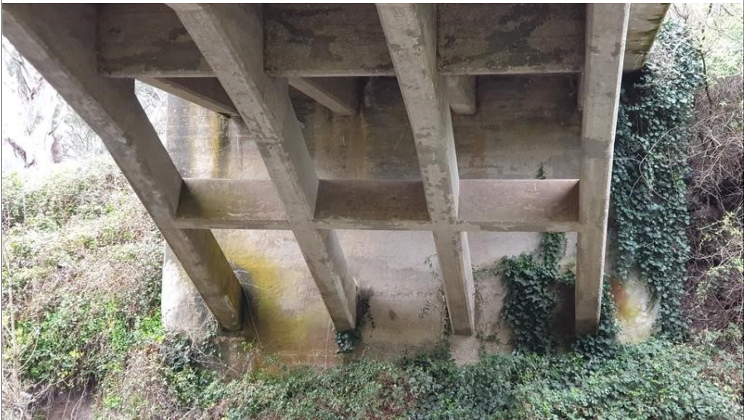
Image Number: 47 Image Name: BR004_047 Description: View of cross bracing.
