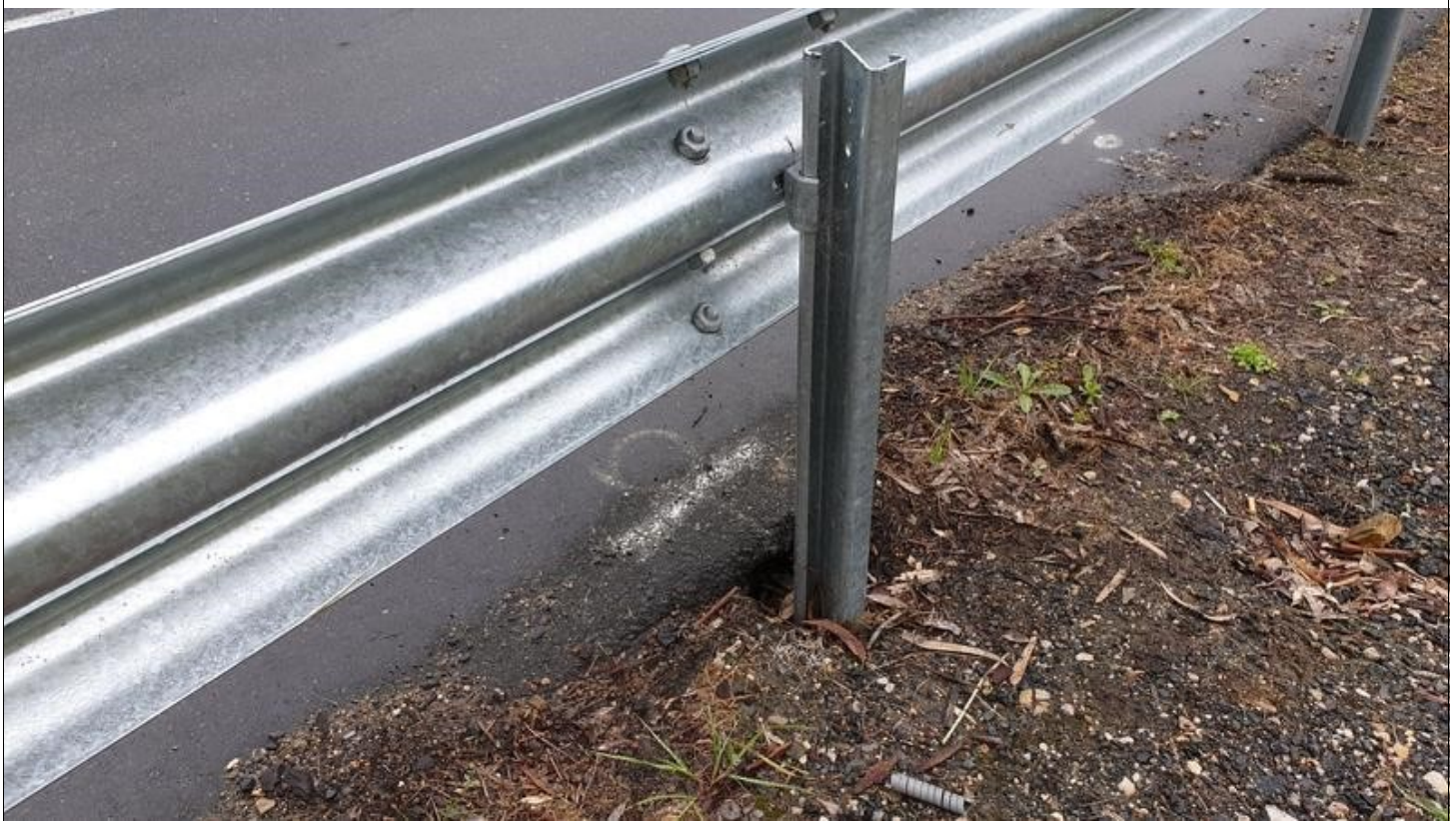
Image Number: 13 Image Name: BR004_013 Description: View of loss of material (200mm) on post on guardrail 2.
