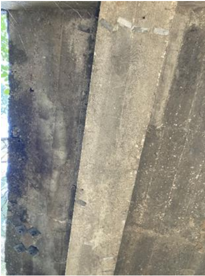
Figure 2.2 Abrasion, delamination and trapped moisture near end 2 of girder 4
