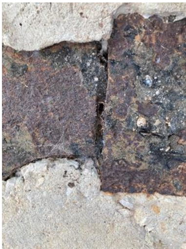
Figure 2.28 Girder 2 corrosion and section split at mid-span
