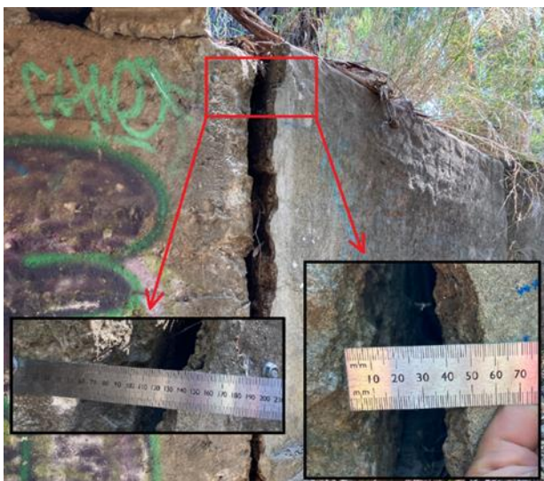
Figure 2.30 40 mm wide gap/separation between abutment 1 and wingwall 1 left-hand side – the spacing of anchorage bolts measured as 200 mm
