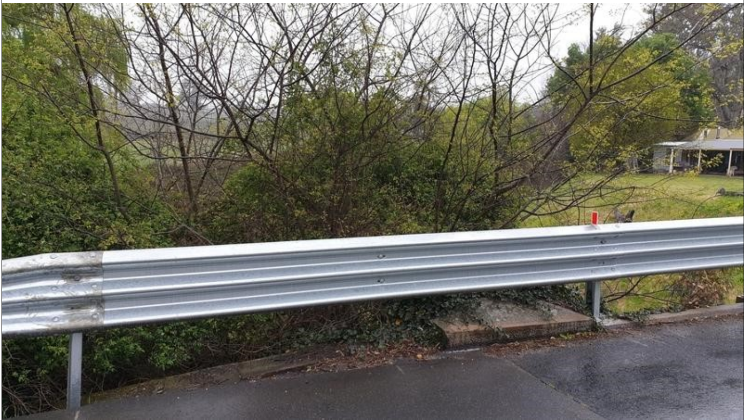
Image Number: 15 Image Name: BR004_015 Description: View of vegetation overgrown encroaching on component on railings/barriers 1.
