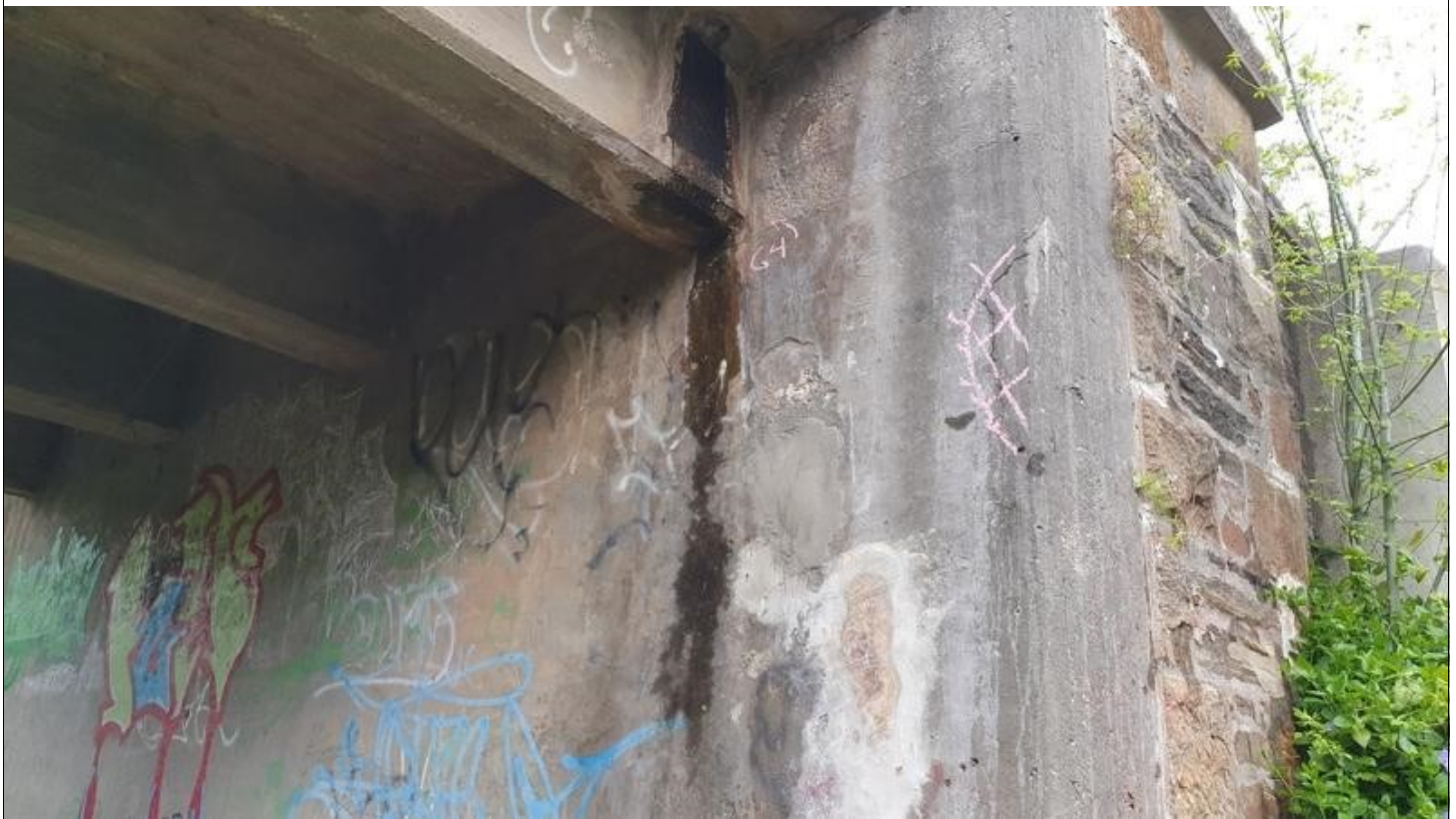
Image Number: 59 Image Name: BR004_059 Description: View of moderate spalling throughout component. Moisture staining under girder 4 on abutment 1.
