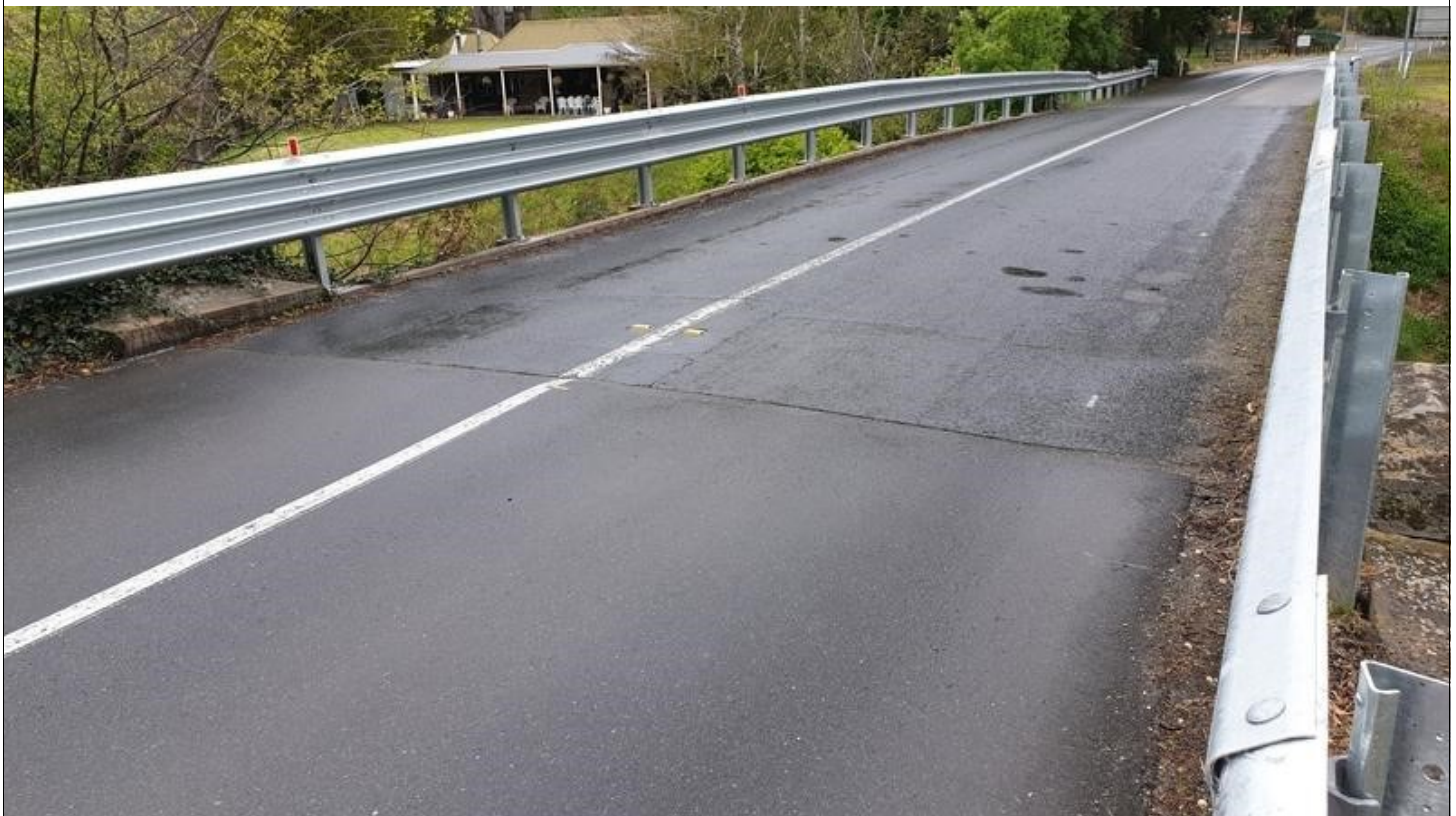
Image Number: 12 Image Name: BR004_012 Description: View of crack coinciding with joint location on bridge approach 1.
