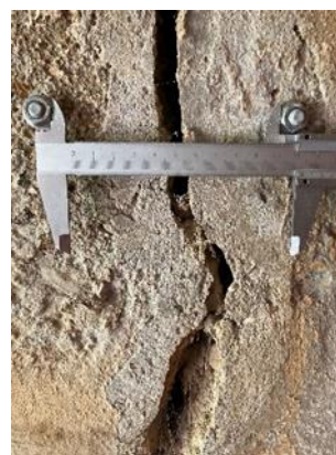
Figure 2.24 Installed anchorage bolts spacing, left-hand side of abutment 1 – 102 mm
