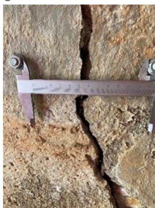
Figure 2.23 Installed anchorage bolts spacing, right-hand side of abutment 1 – 120 mm
