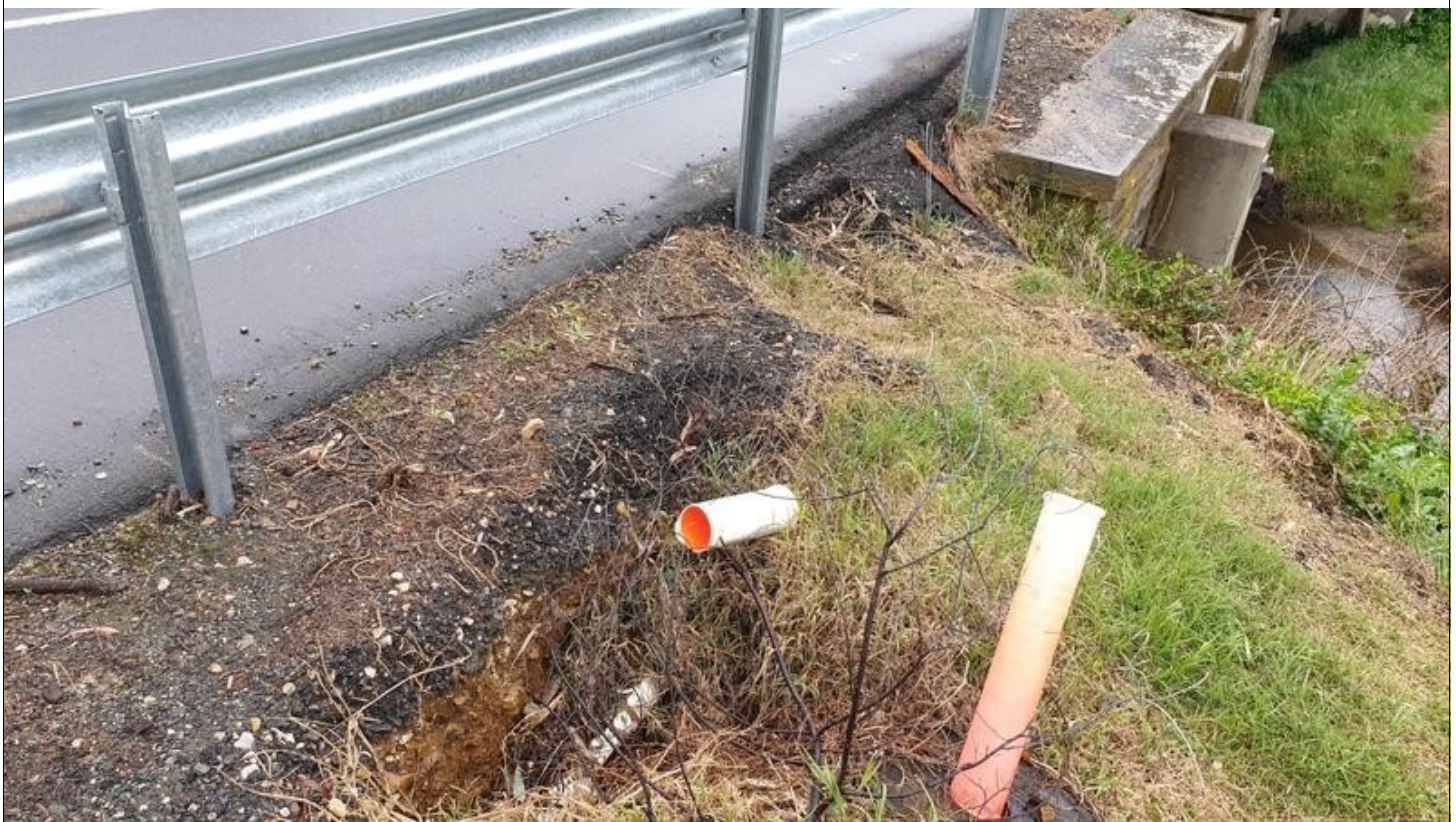
Image Number: 11 Image Name: BR004_011 Description: View of erosion of soil exposing utilities below on bridge approach 1.
