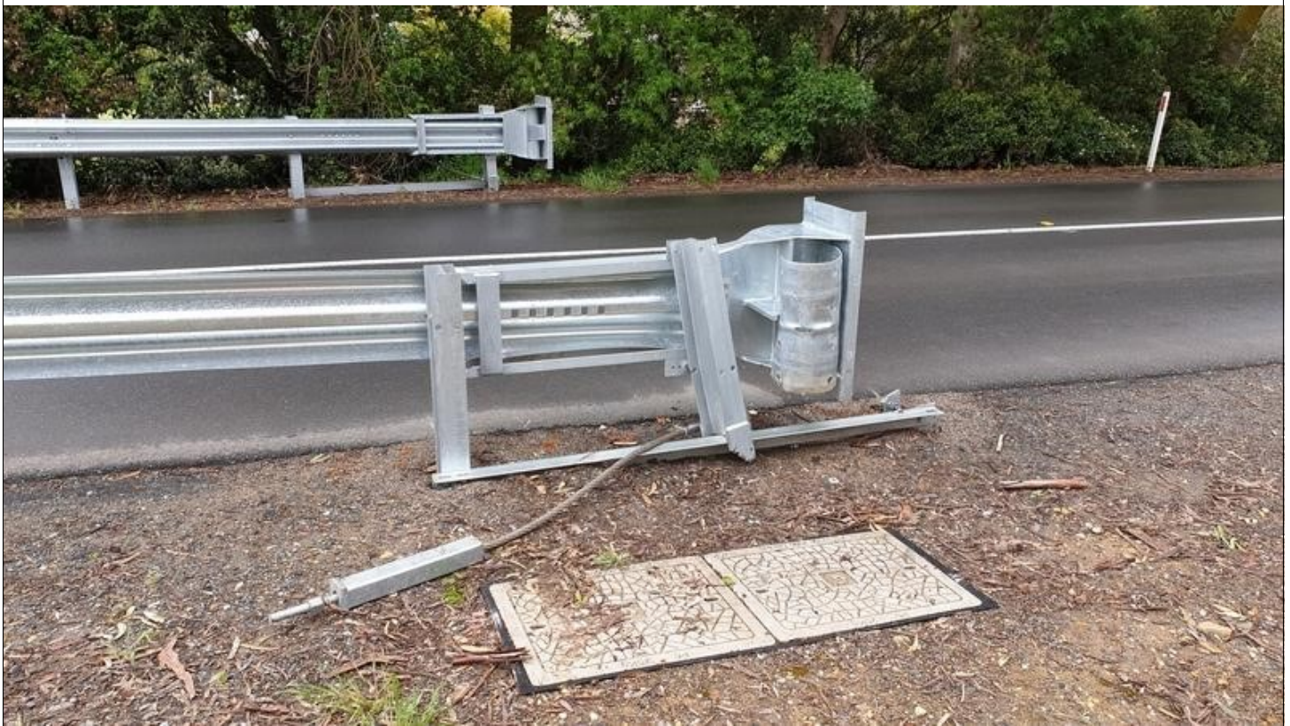
Image Number: 33 Image Name: BR004_033 Description: View of tensioner and post not connected on terminal on guardrail 2.
