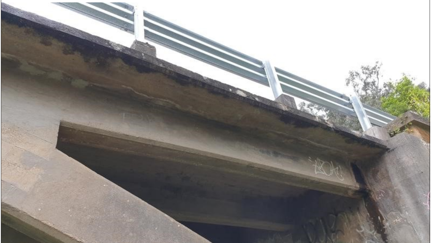
Image Number: 41 Image Name: BR004_041 Description: View of moisture staining throughout deck edges on deck slab 1.
