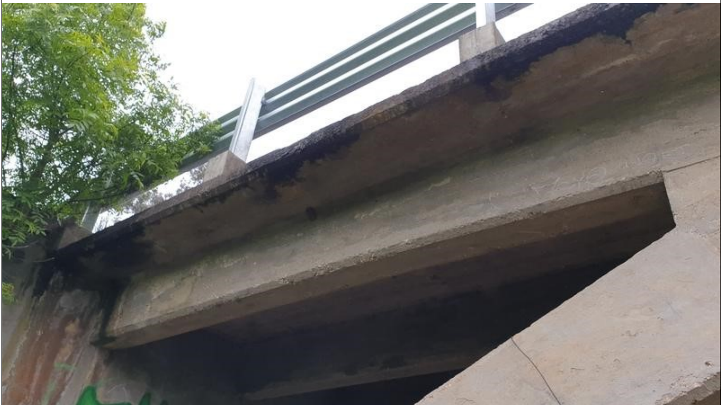
Image Number: 44 Image Name: BR004_044 Description: Additional view of moisture staining throughout deck edges on deck slab 1.
