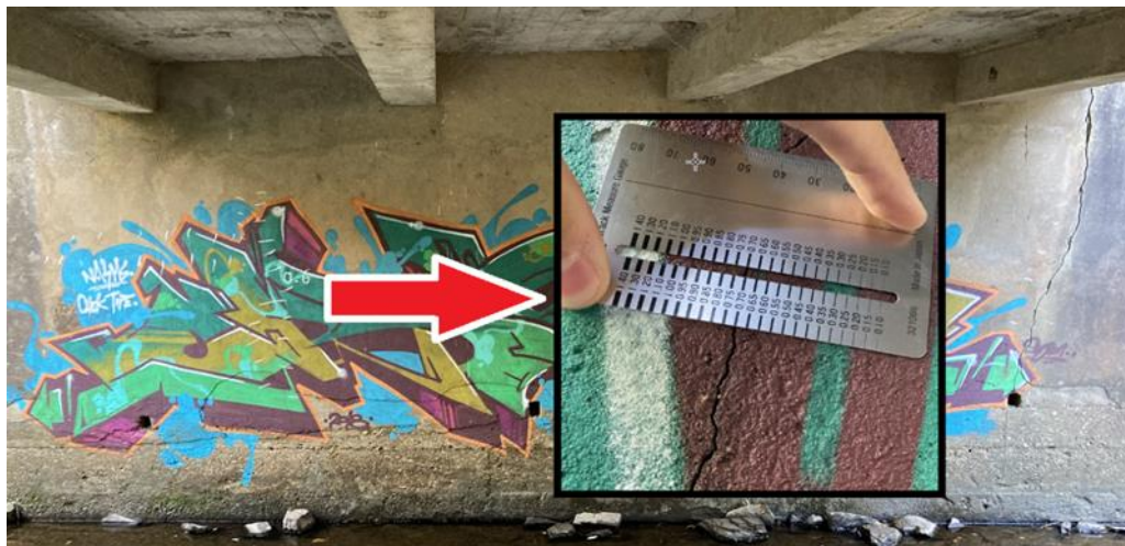
Figure 2.8 Moderate 0.7 mm wide vertical crack at right-hand side of abutment 1 (under girder 3) extending 2 m from the soffit
