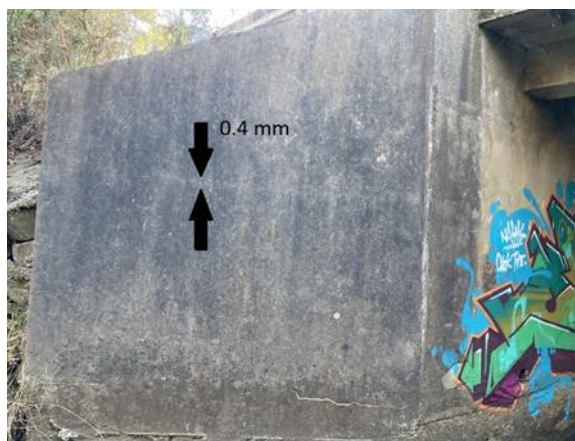
Figure 2.11 Moderate 0.4 mm wide horizontal crack extending across wingwall 1 right-hand side
