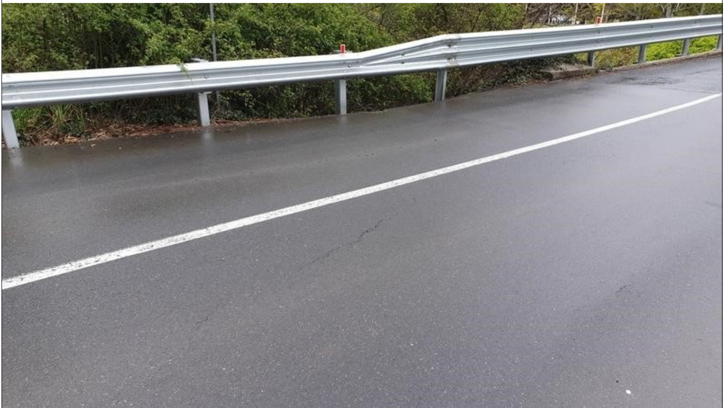
Image Number: 9 Image Name: BR004_009 Description: Additional view of minor Cracking on wearing surface on bridge approach 1.
