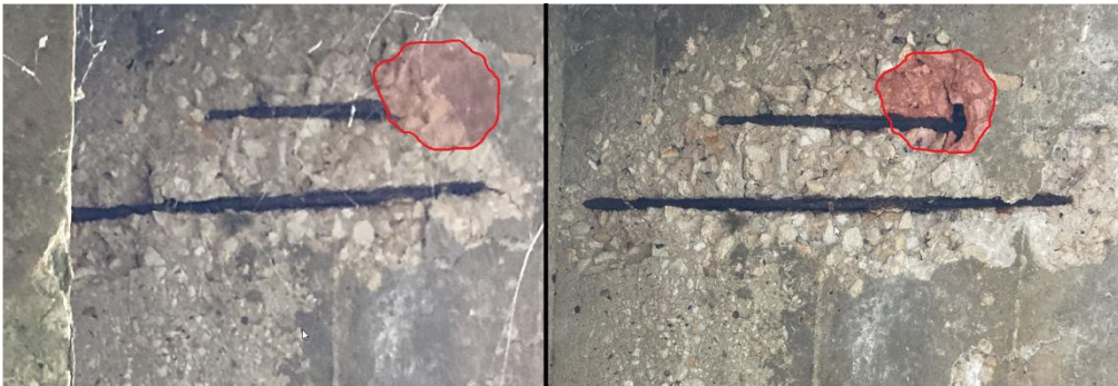
Figure 2.13 Example of before (left) and after (right) applying sounding hammer – located near end 2 of girder 1
