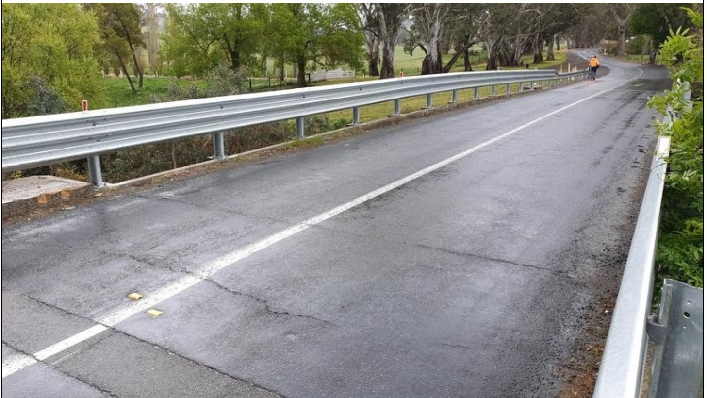
Image Number: 23 Image Name: BR004_023 Description: View of minor rutting and cracking throughout component on wearing surface 1.
