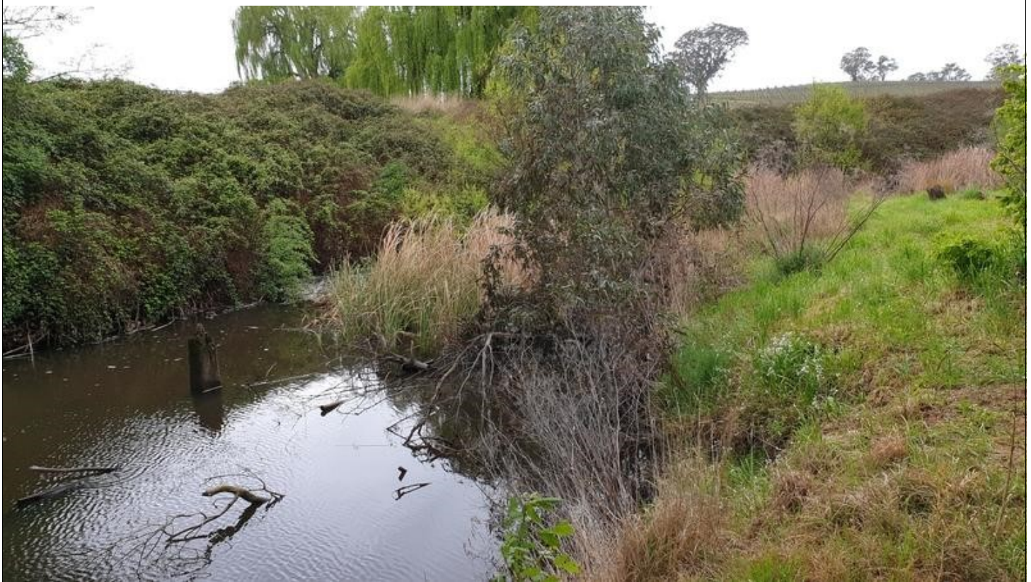
Image Number: 67 Image Name: BR004_067 Description: View of vegetation obstructing waterway on left hand side on waterway 1.
