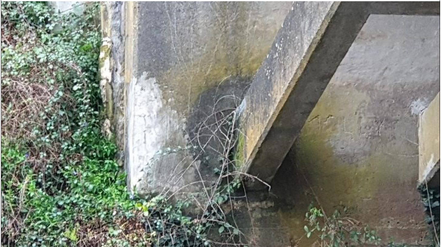
Image Number: 38 Image Name: BR004_038 Description: View of efflorescence noted near column 4 on abutment 1.
