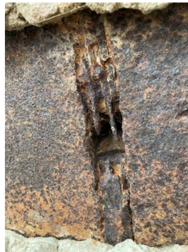
Figure 2.29 Girder 4 corrosion and section split at mid-span
