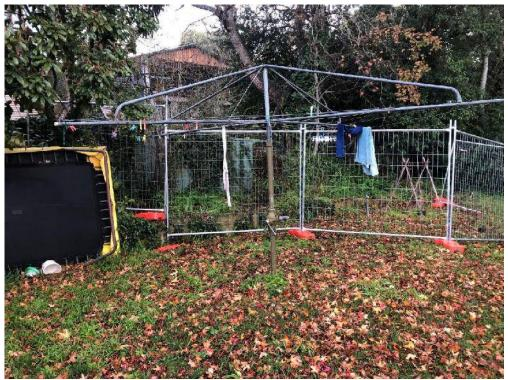
Figure 14-15: Temporary fence installed to secure the area before it was backfilled.
