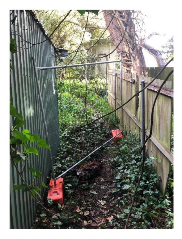
Figure 16: Temporary fence installed to secure the area before it was backfilled.
