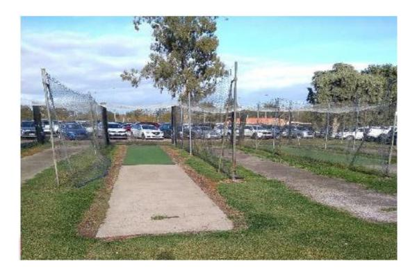
Following Development Approvals consent from the Adelaide Hills Council (AHC), the project commenced with club members removing the old nets and posts, followed by groundwork, base, and levelling. Initial infrastructure installed posts for the fencing and nets, the concrete pad being poured and the chain link fence installed.
