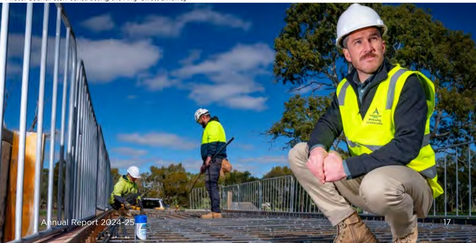
Photo: Council staff constructing the Amy Gillett Bikeway
