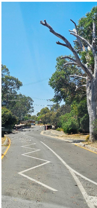
Photo 6 Council Road – Fairview Road – Emu Crossing from other direction, zig zag line marking and no parking line marking in place.
