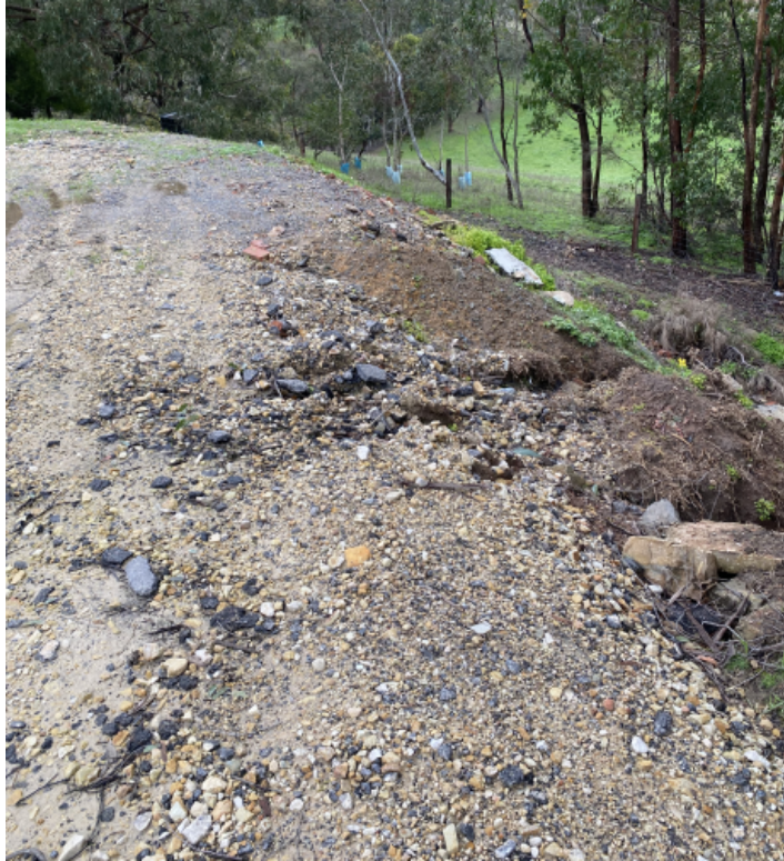
NEW BATTER INTEFACE WITH PREVIOUS FILL BATTER (VEGETATED)
