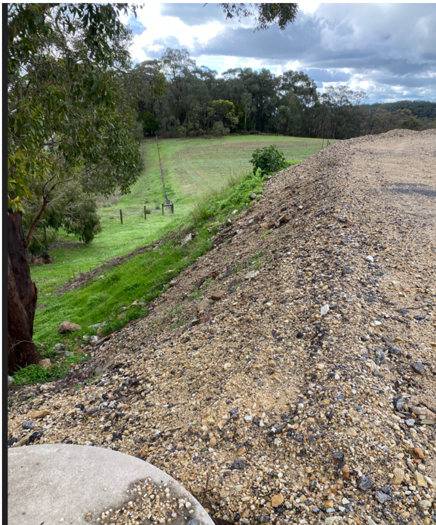
NEW BATTER INTEFACE WITH PREVIOUS FILL BATTER (VEGETATED)
